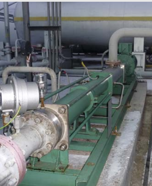
NM105SY Capacity: 44-94 m 3 /h Pressure: 18 bar Medium: multiphase water, gas, crude oil, H 2 S Gas rate: 85%
