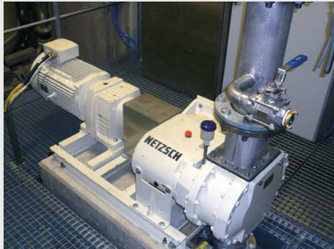
The TORNADO® T1 in use in a paper mill. Kaolin tankers are unloaded at 75 m 3 /h against a pressure of up to 4 bar.
