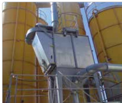
INSTALLATION ON TOP OF CEMENT WEIGH HOPPER
