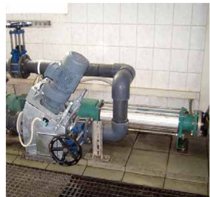
A strong team offers process reliability and efficiency: M-Ovas® and NEMO® progressing cavity pump
