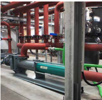
The NEMO® progressing cavity pump: an energy-efficient solution for high pressure ranges too
